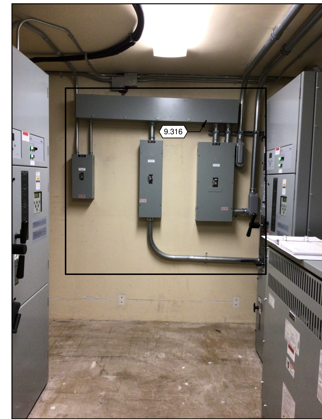
4 EXISTING WIREWAY AND ENCLOSED BREAKERS - 1 NO SCALE
