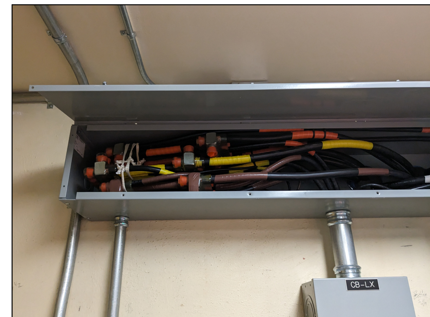
5 EXISTING WIREWAY AND ENCLOSED BREAKERS - 2 NO SCALE
