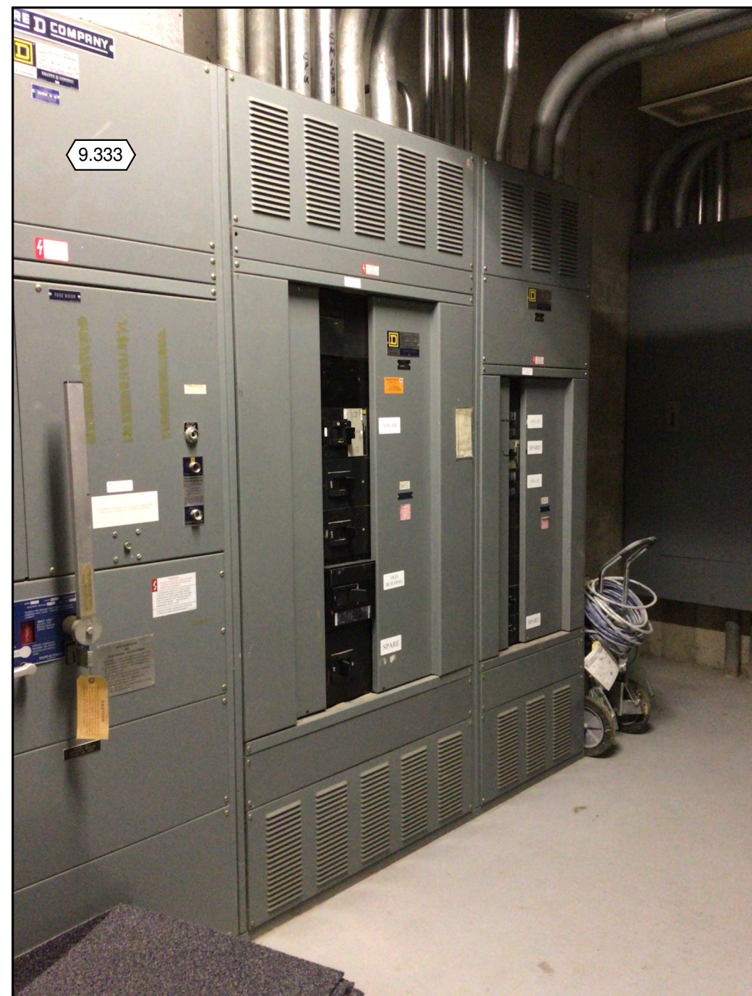
1 EXISTING SWITCHBOARD MSB NO SCALE
